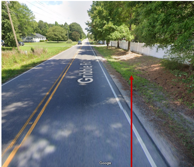
c) Existing Stormwater Swales Along Gribble Road
