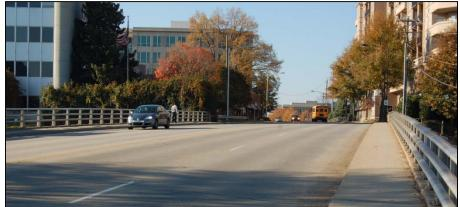
Though most pedestrians prefer separation between sidewalks and travel lanes, bridges often create obstacles for pedestrian travel because of a lack of dedicated facilities. Sidewalks located directly adjacent to travel lanes provide a dedicated facility for pedestrian travel along roadways with lower traffic volumes and speeds.
