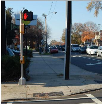
Pedestrian signals should be placed in locations that are easily seen from across an intersection and nearby curb ramps. This location provides access to the pedestrian actuated button (if available) and accurate guidance to the visually impaired for signals with auditory warnings.
