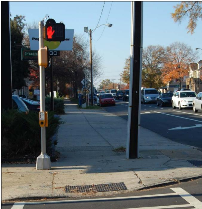
**Pedestrian signals should be placed in locations that are easily seen from across an intersection and nearby curb ramps. This location provides access to the pedestrian actuated button (if available) and accurate guidance to the visually impaired for signals with auditory warnings.**
