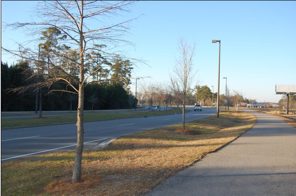
**This landscape buffer along Harrelson Boulevard provides separation for cyclists and pedestrians from the travel lane. It is also used as a temporary detention area for storm water runoff during rain events.**
