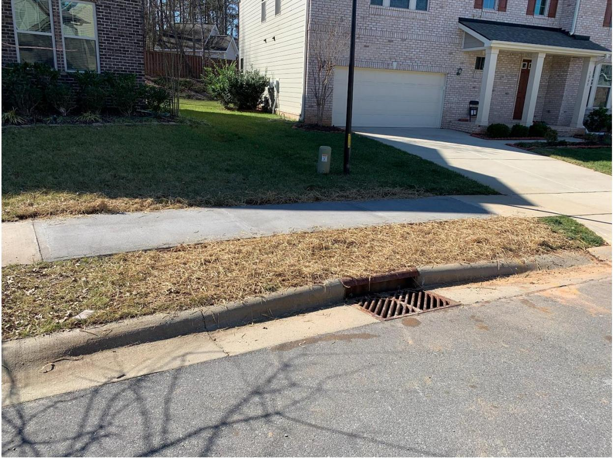
2. 4208 Gold Crest Drive (Golden Acres) – The ditch line in front of this property needed to be regraded and the galvanized steel driveway pipe was replaced with a reinforced concrete pipe.
