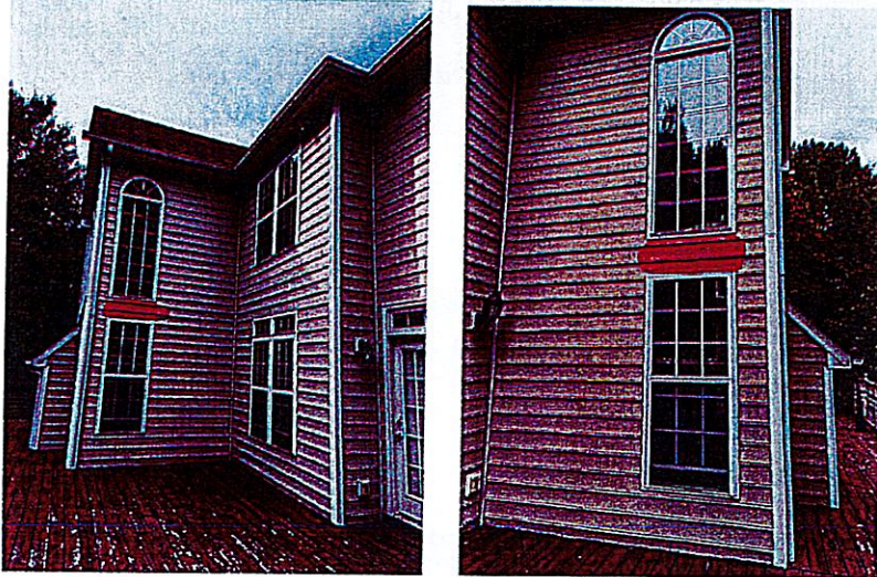
Figure 5: Architecture of house showing inability to put a roof between the two vertically stacked windows on either side of the outset on the rear of the house:
