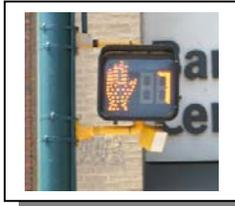
**Countdown signals** are pedestrian signals that show how many seconds the pedestrian has remaining to cross the street. The countdown can begin at the beginning of the WALK phase, perhaps flashing white or yellow, or at the beginning of the clearance, or DON'T WALK phase, flashing yellow as it counts down.
