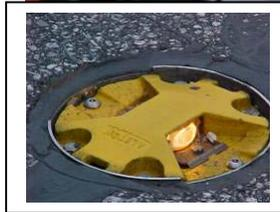
**In-pavement flashing warning light system**
